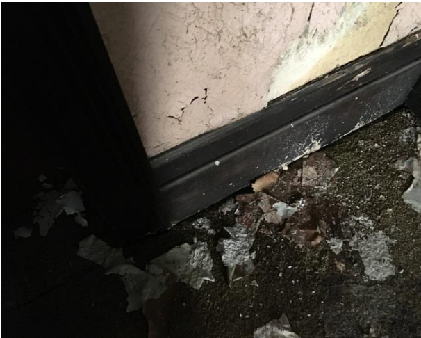
PICTURE 27 – INTERNAL VIEW OF SKIRTING.
