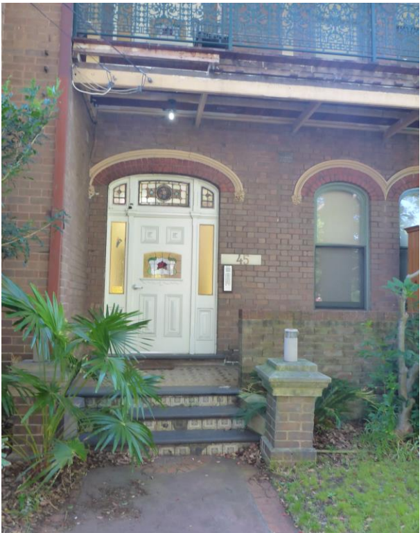
PICTURE 35 – DETAIL LOWER GROUND LEVEL FRONT FAÇADE.
