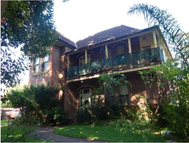
PICTURE 33 – PRINCIPAL EASTERN FAÇADE.
