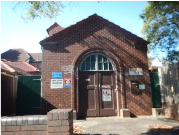
PICTURE 11 – HERITAGE LISTED SUBSTATION AT 2B COOPER STREET
