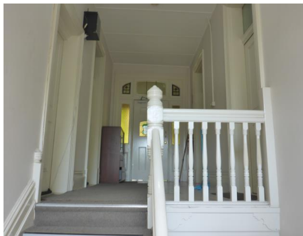
PICTURE 38 – INTERNAL VIEW
