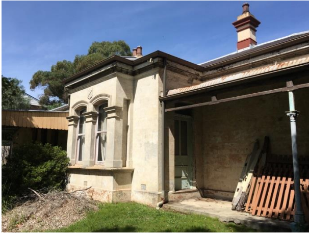
PICTURE 21 – EXTERNAL VIEW OF EASTERN BAY.
