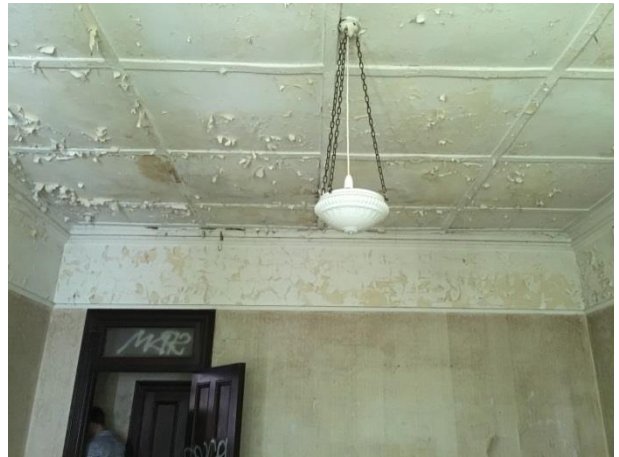
PICTURE 26 – INTERNAL VIEW OF PRINCIPAL ROOM AND TIMBER JOINERY.
