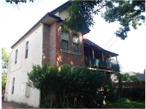
PICTURE 34 – PRINCIPAL EASTERN FAÇADE.
