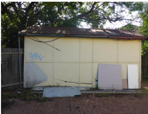
PICTURE 37 – EXTERNAL VIEW
