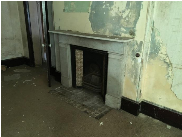
PICTURE 25 – INTERNAL VIEW OF PRINCIPAL ROOM.
