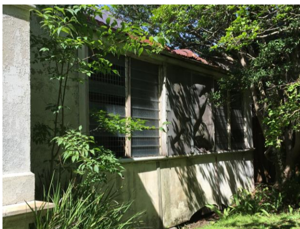
PICTURE 20 – EXTERNAL VIEW OF INFILLED WESTERN FAÇADE.
