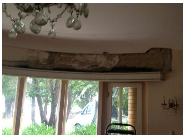
PICTURE 41 – INTERIOR OF CURVED FRONT SECTION OF THE HOUSE
