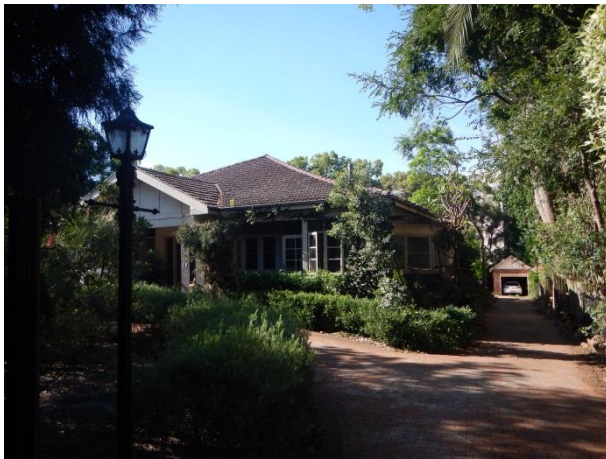
PICTURE 3 – EARLY TWENTIETH CENTURY DWELLING AT 16-18 COOPER STREET
