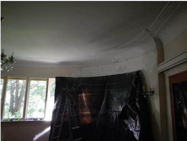
PICTURE 49 – INTERNAL VIEW
