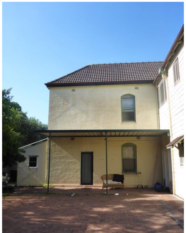
PICTURE 36 – NORTHERN FAÇADE.
