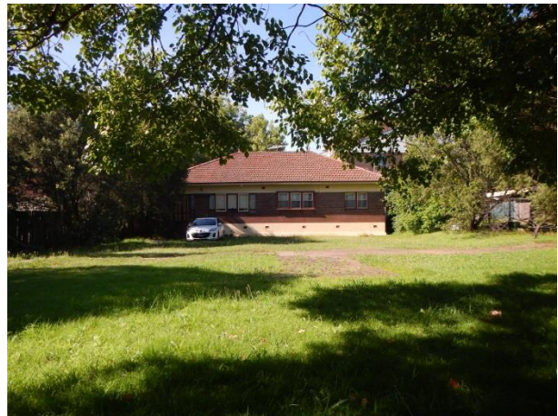
PICTURE 12 – MID TWENTIETH CENTURY DWELLING AT 2A COOPER STREET
