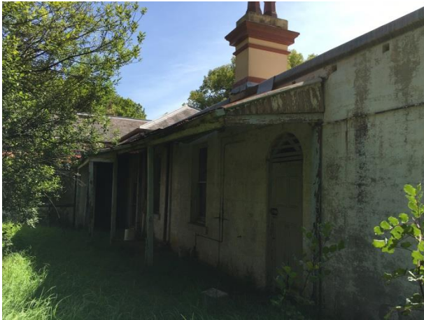
PICTURE 23 – EXTERNAL VIEW OF WESTERN FAÇADE.
